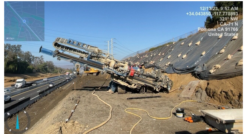
Retaining wall 131, verification soil nail drilling.
