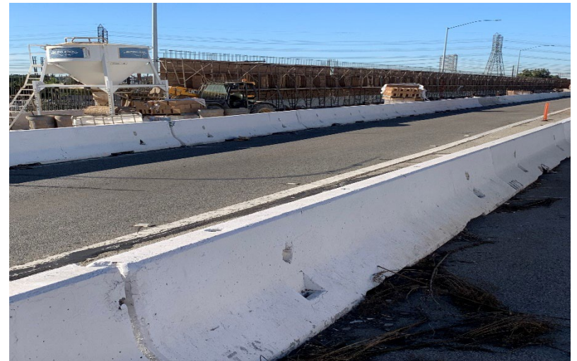
SB 405 Crenshaw Blvd off ramp (SW #815)
