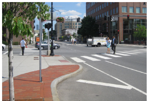
Curb extension and crosswalk
