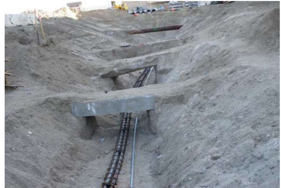
Underground utility work
