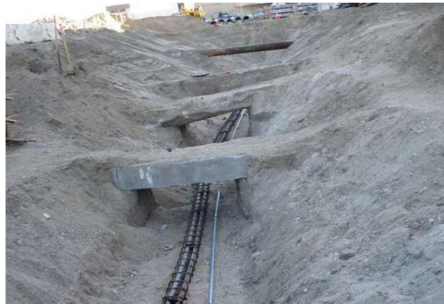
Underground utility work
