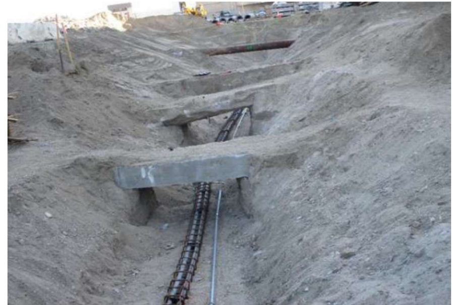
Underground utility work
