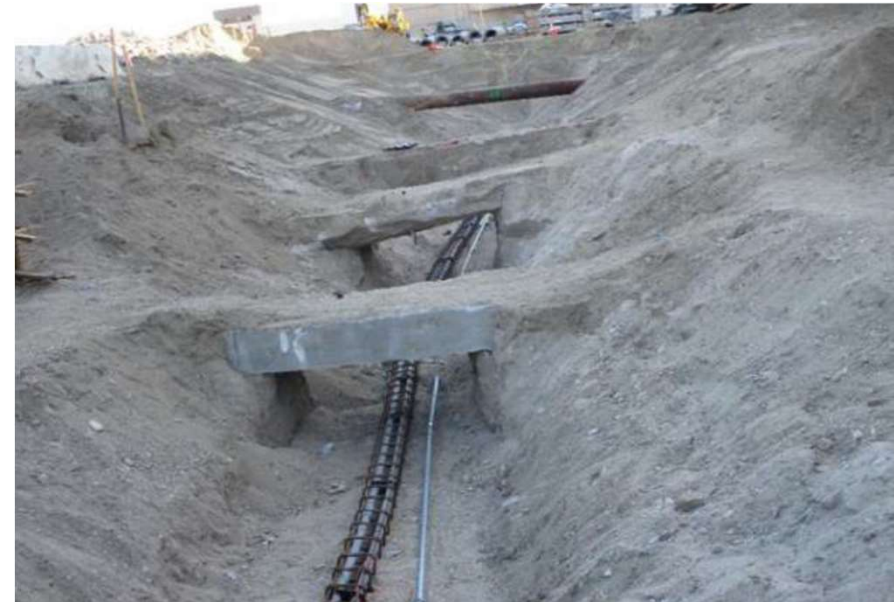
Underground utility work
