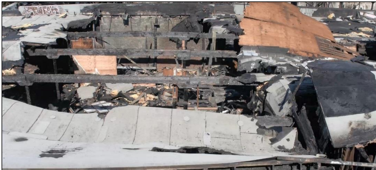
Figure 7. Citizens Warehouse/Lysle Storage Company (Pickle Works). Drone footage of southern portion. Looking north, northeast, and downward. Zephyr UAS: November, 2018.
