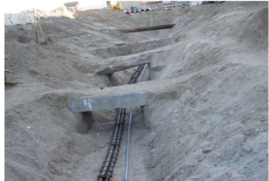
Underground utility work
