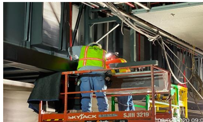
MARTIN LUTHER KING JR. STATION – Installing edge lighting at the plaza level
