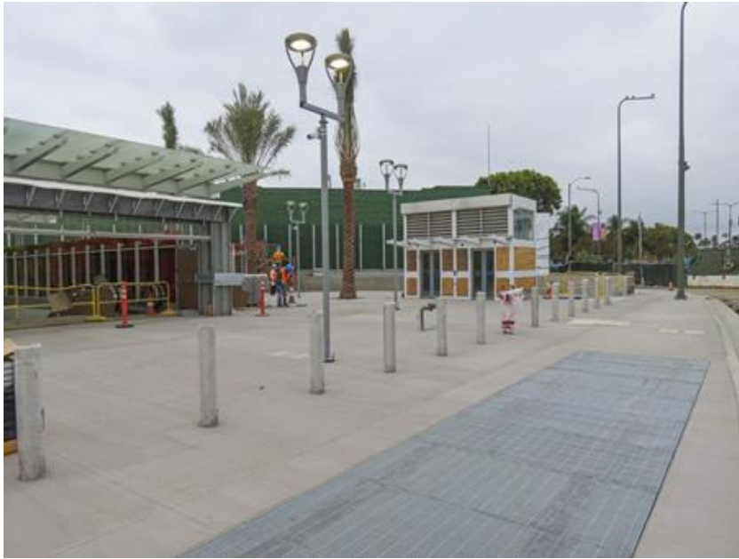
Leimert Park Station – plaza, lighting, landscaping, bollards, elevator and main entrance
