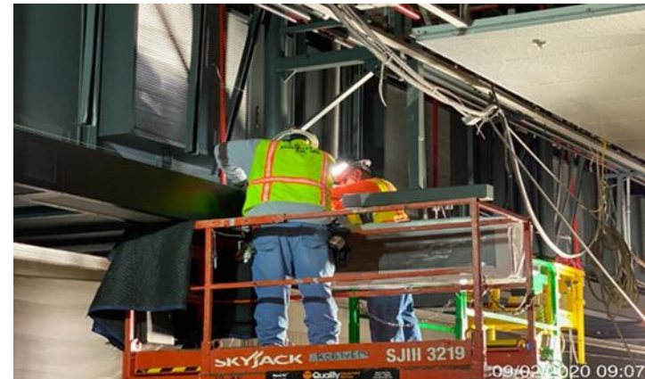
MARTIN LUTHER KING JR. STATION – Installing edge lighting at the plaza level
