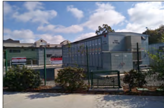
Photo ES-7: Typical TPSS for LRT
