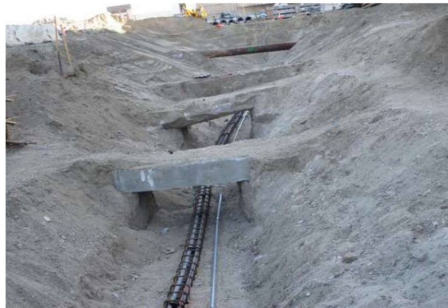
Underground utility work
