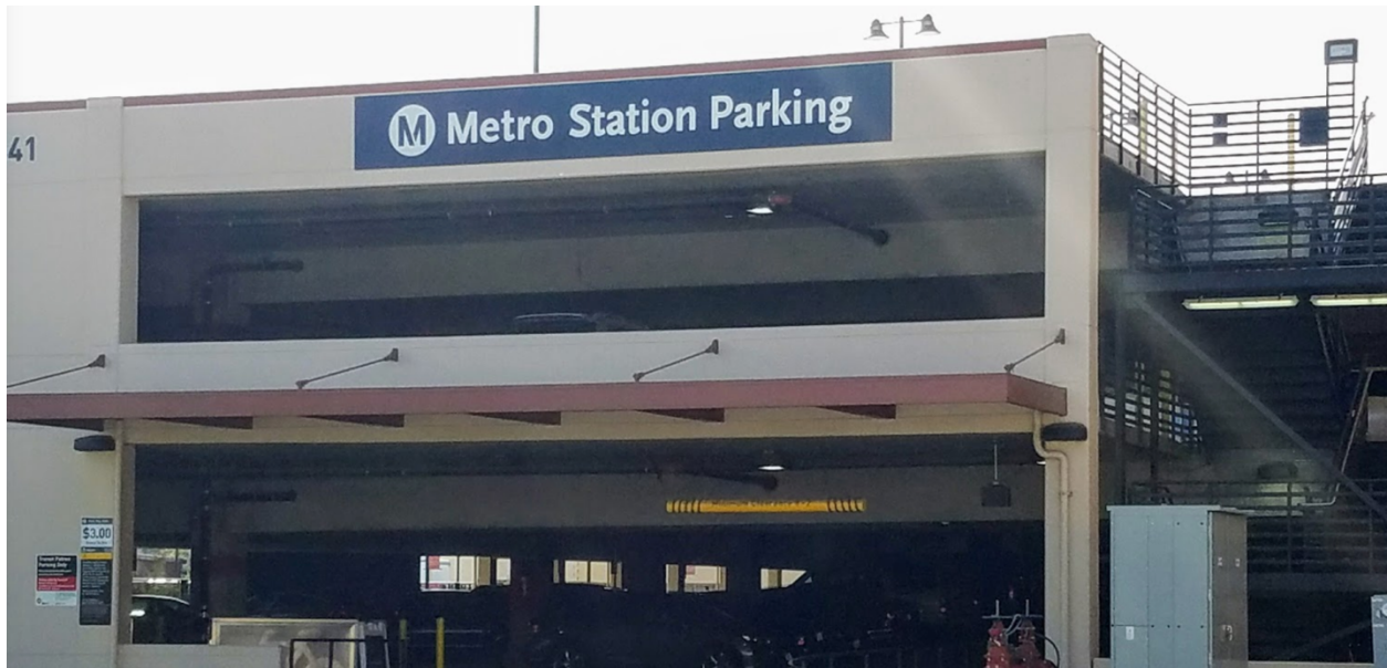
Figure 4.10.7 Monrovia Parking Garage (view from Primrose Avenue)
