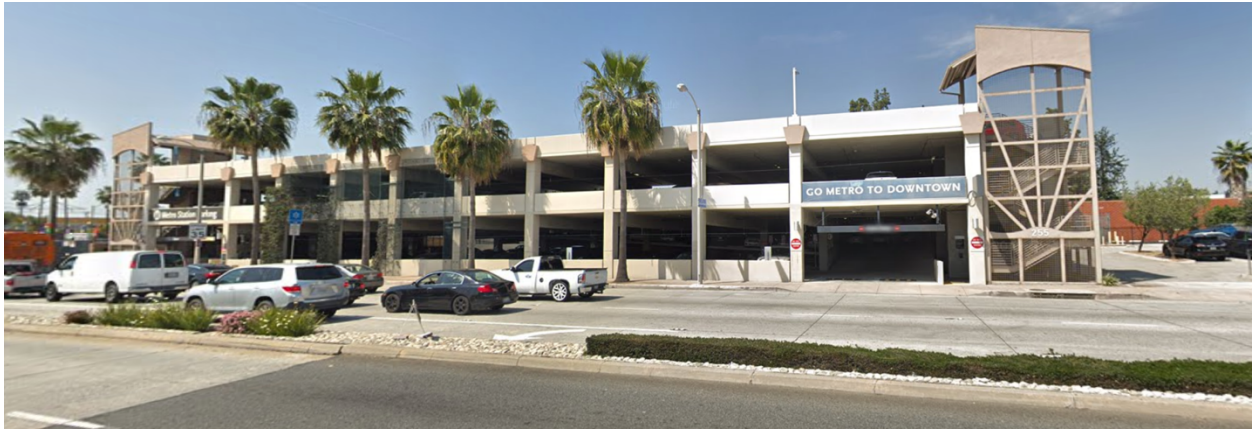
Figure 4.10.2 Atlantic Parking Garage (view from Atlantic Boulevard)
