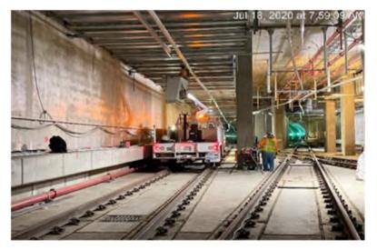
Continue installing supports and fixtures for the crossover lighting at the invert level of Expo/Crenshaw Station.
