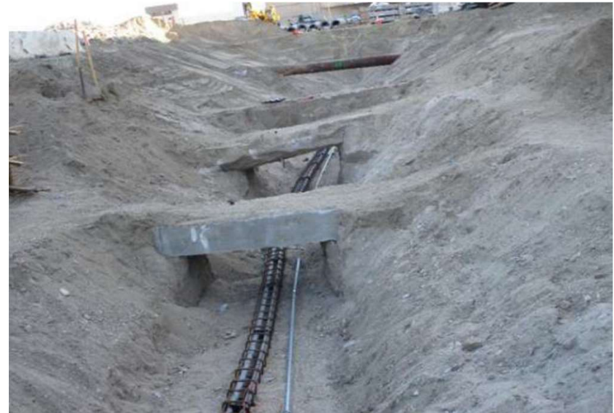
Underground utility work
