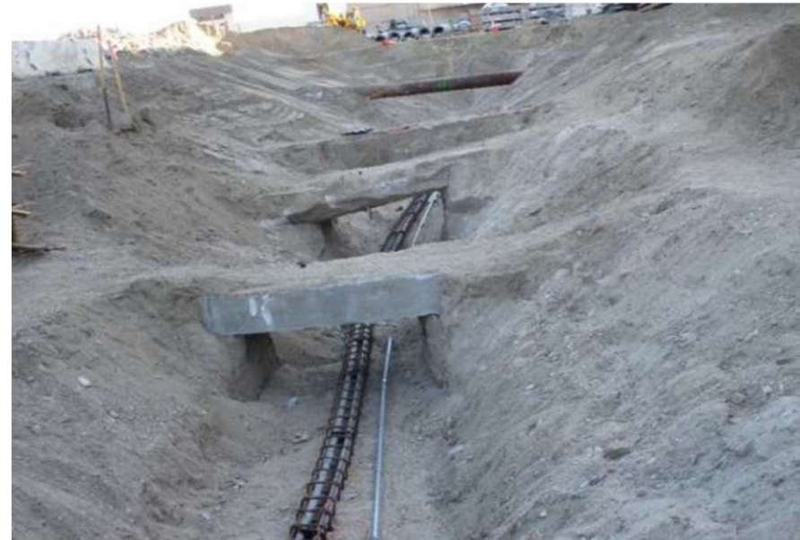
Underground utility work
