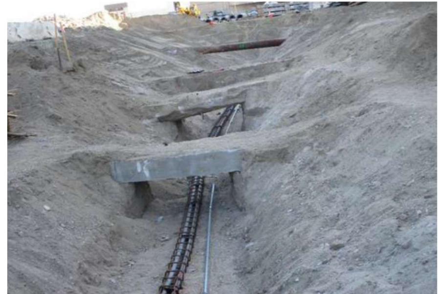
Underground utility work
