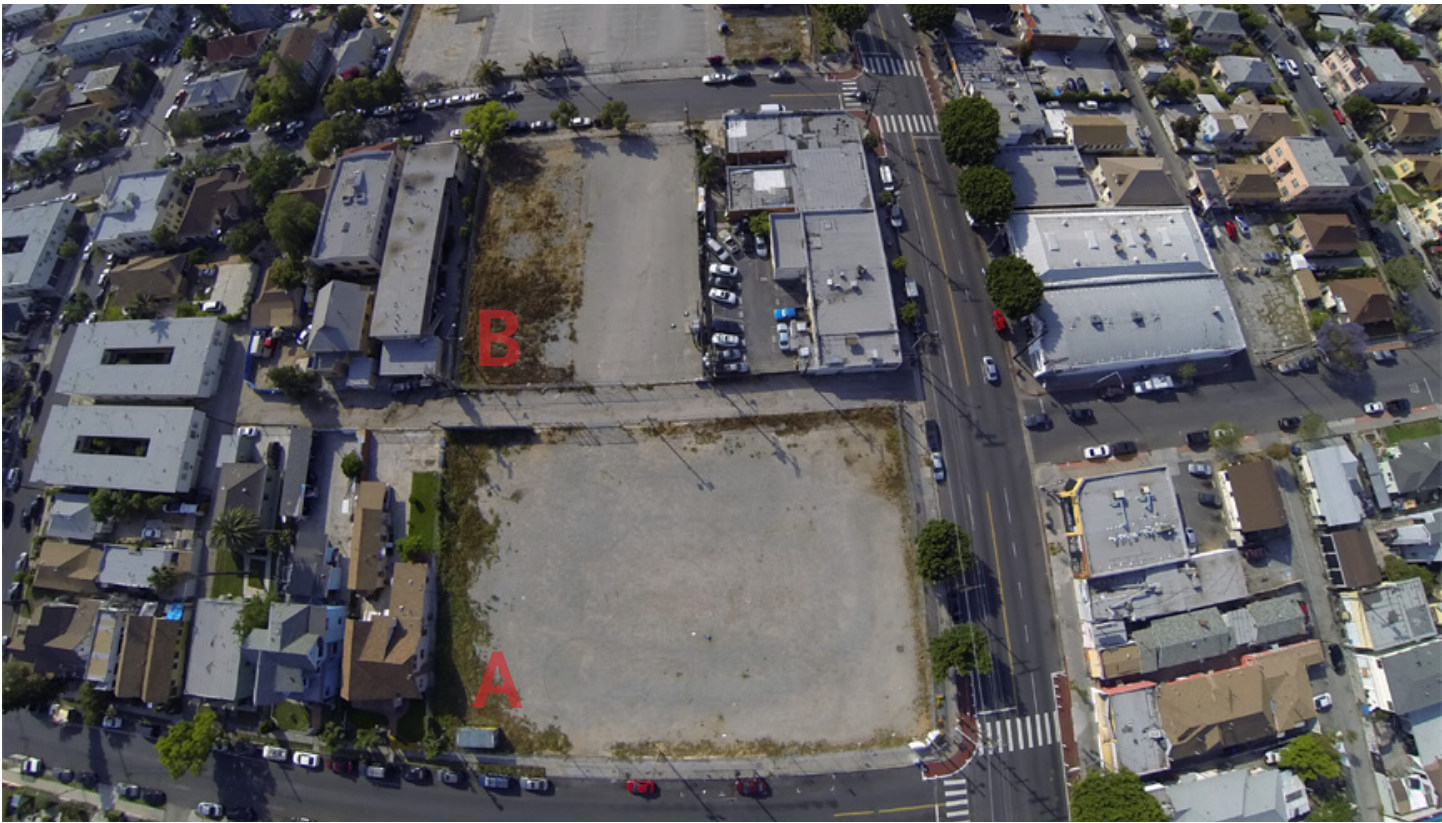
Aerial Photo of Existing Conditions, 2016
