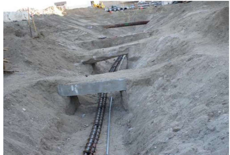
Underground utility work
