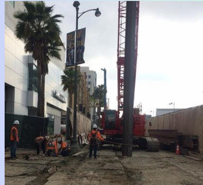
C1045 Contractor Installing Pile at Wilshire/La Brea Station
