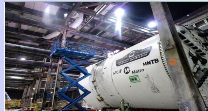
Start of TBM assembly in Expo/Crenshaw Station
