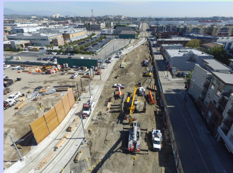
Shoofly installation at 1 st Street
