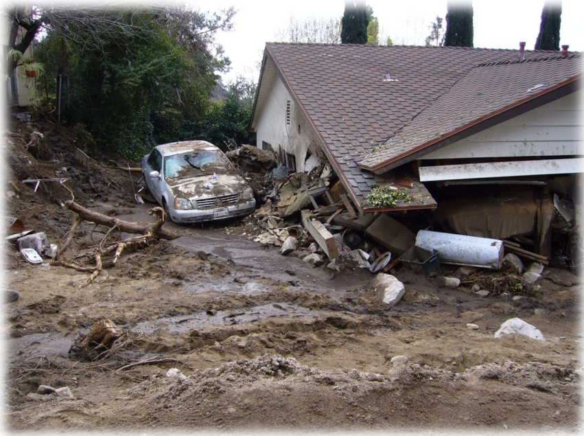
Caption: House damaged by debris flows generated in Mullally Canyon in response to a rainstorm on February 6, 2010. The drainage basin above this home was burned the previous summer by the Station Fire, which was the largest fire in the history of Los Angeles County at the time.
