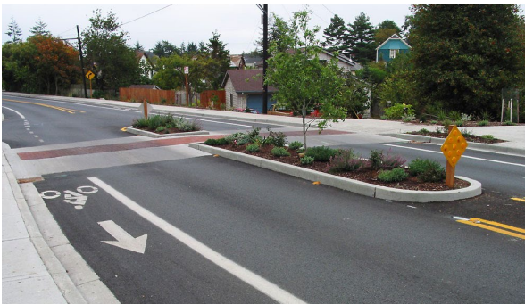
Class II Bicycle Lane (Dedicated On-Street)
