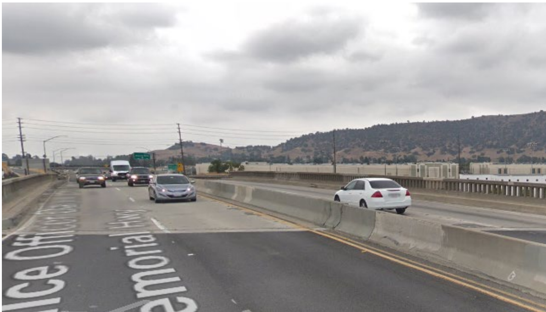
BEFORE RAIL BRIDGE RECONSTRUCTION
