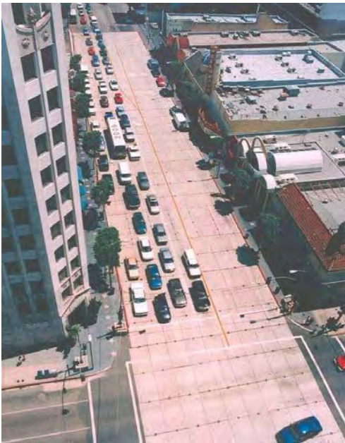
Figure 3-1: Roadway Operations Restored on Temporary Decking System
