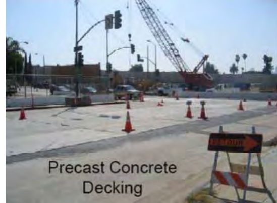
Figure 3-4 Precast Concrete Decking
