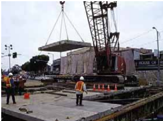
Figure 3-4: Installation of Decking (1 of 2)
