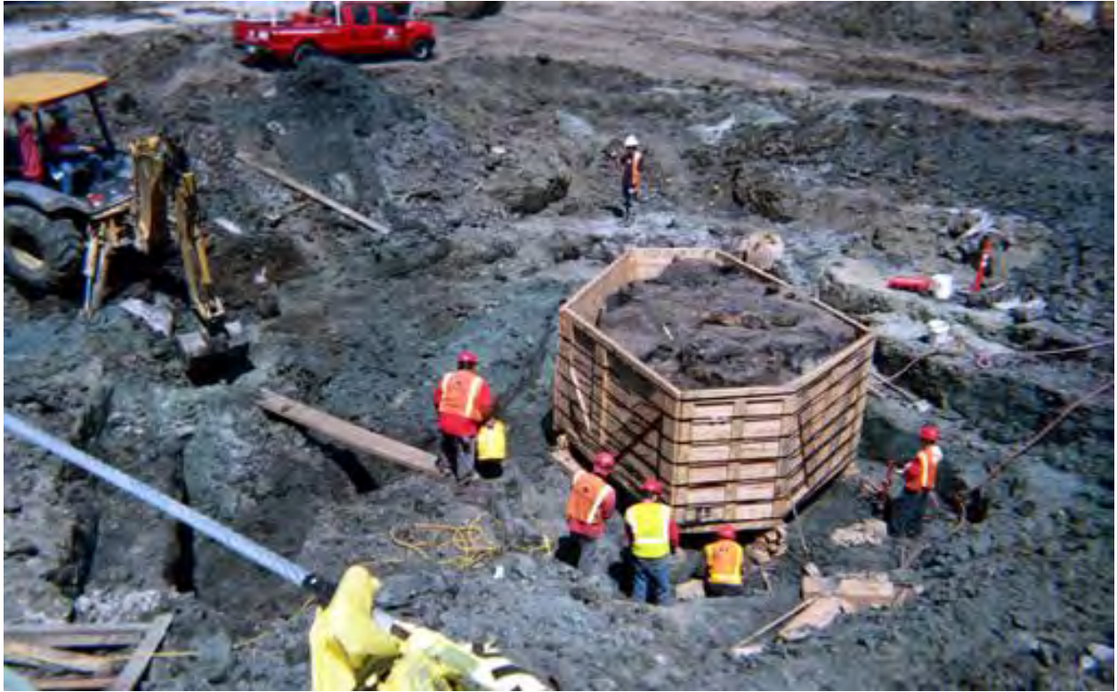
Fig 9: Secure the tree box with metal bands
