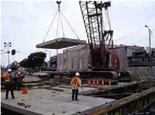
Figure 3-4: Installation of Decking (1 of 2)
