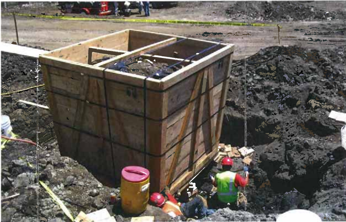
Fig 10: Tunnel under the tree box
