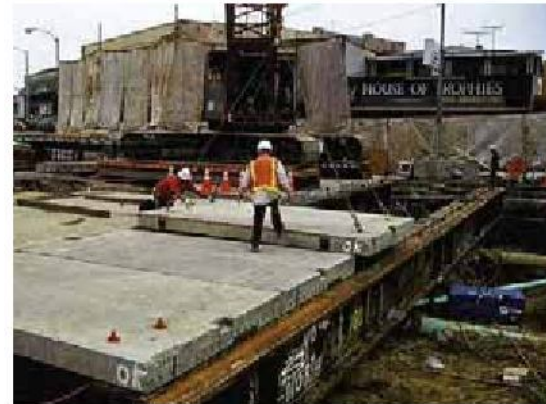
Figure 3-5: Installation of Decking (2 of 2)
