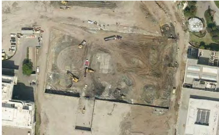
Figure 4-20: Aerial View of Project 23 Excavation with Dark Tar Seeps
