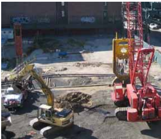
Figure 3-14: Slurry Wall Construction Equipment
