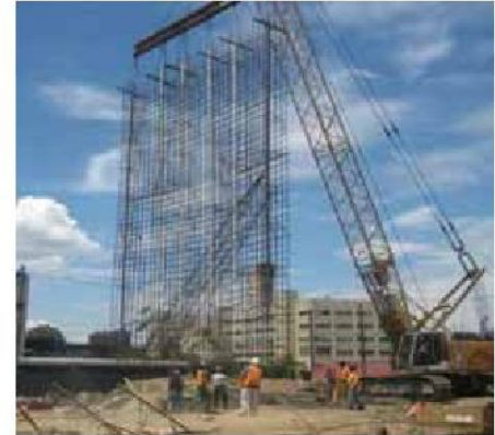
Figure 3-13: Steel Reinforcement Cage for Slurry Wall
