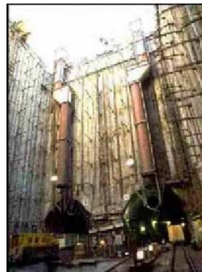
Figure 3-12: Secant Pile Wall at Barnsdall Shaft on Metro Red Line
