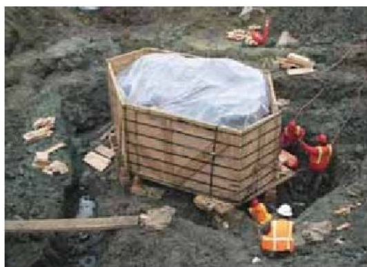
Figure 4-2: Fossil Box Construction at Project 23
