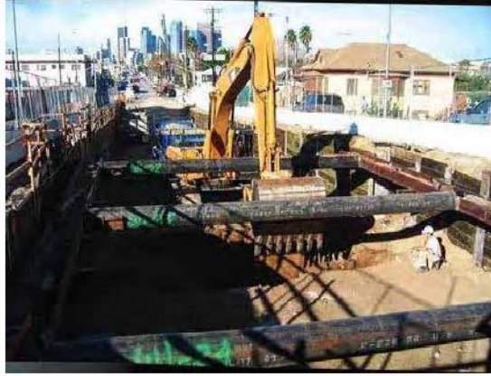
Figure 4-12: Hydraulic Excavator between Struts
