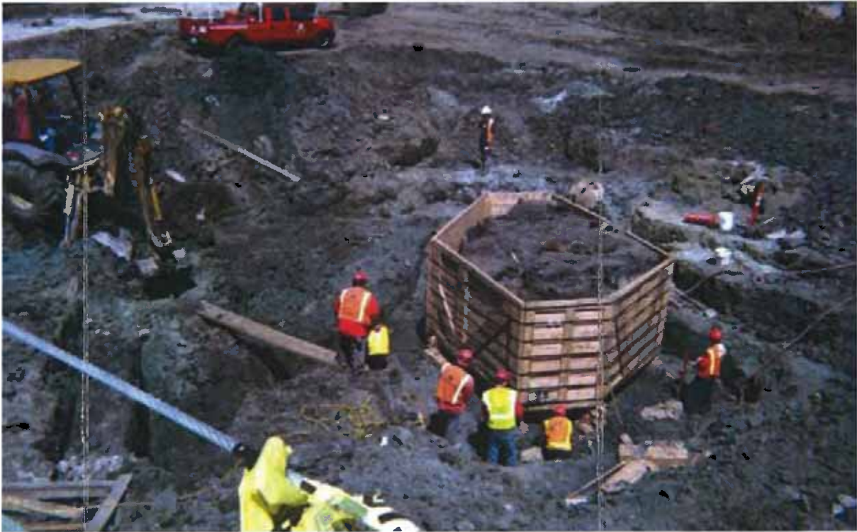
Fig 9: Secure the tree box with metal bands
