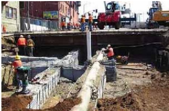
Figure 3-19: Backfilling Utilities in Final Location beneath Road Surface
