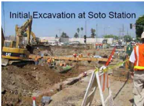
Figure 3-2: Initial Excavation at Soto Station
