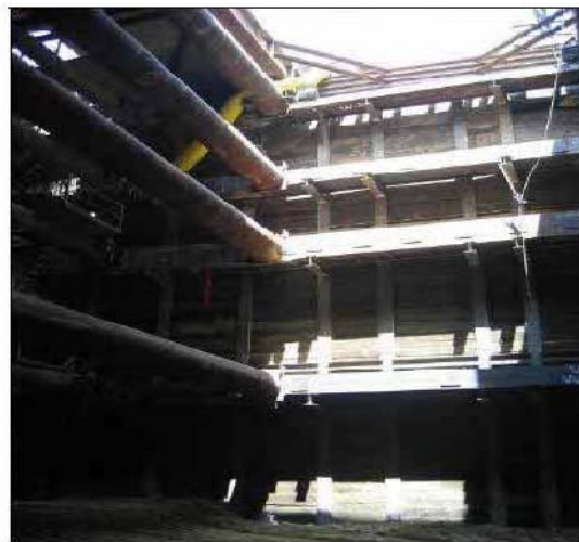
Figure 3-9: Soldier Pile and Lagging
