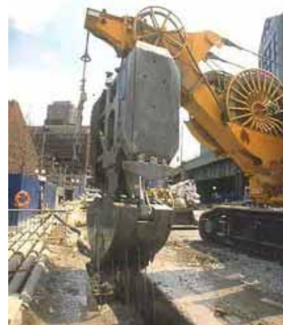
Figure 3-15: Clamshell Digger for Slurry Wall Construction
