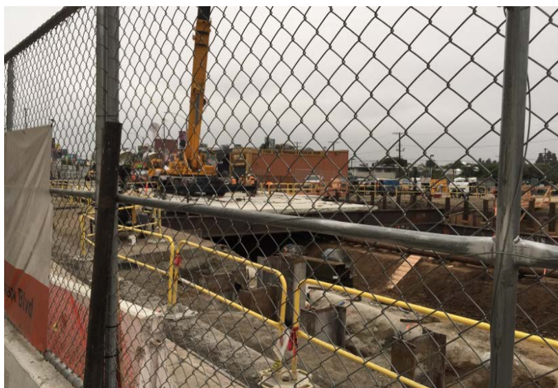
Construction impact from the view of BIF Grantee Dave Velazquez of Dave's Tattoos, 4343 Crenshaw Blvd.
