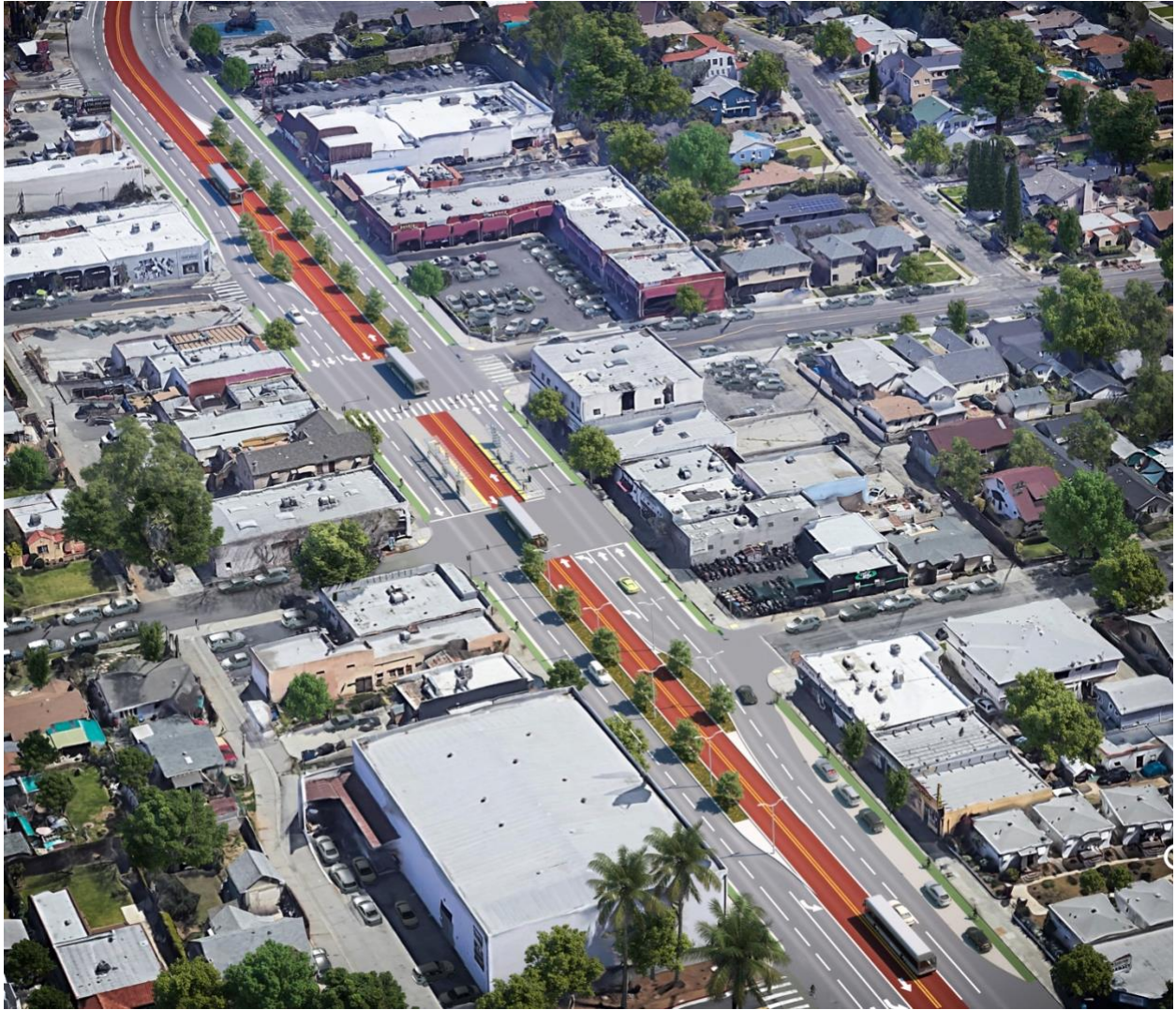
Figure 9: Center-running BRT on Colorado Boulevard in Eagle Rock (east of Eagle Rock Boulevard) – design option maintaining all travel lanes
