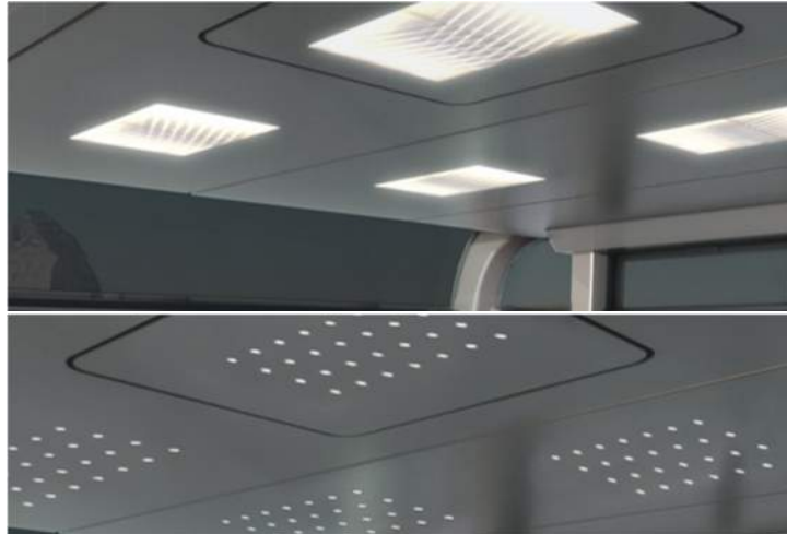
Image 32 – Examples of Interior Lighting
