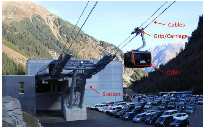
Image 2 – Components of a 3S Gondola System
