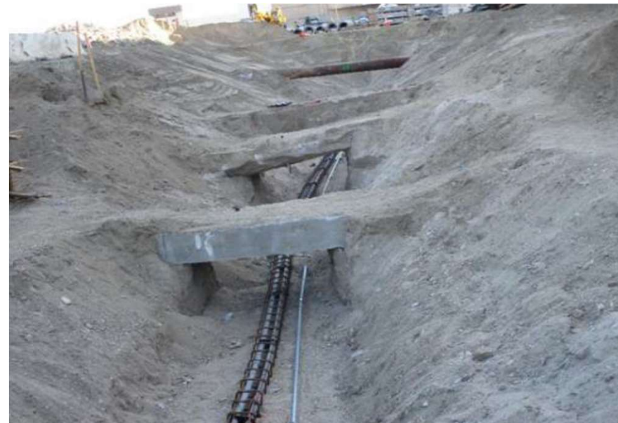
Underground utility work
