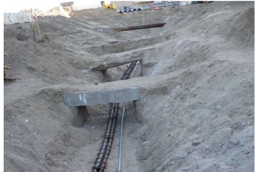
Underground utility work
