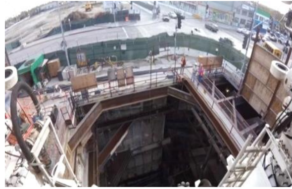
Example of a Construction Staging Site
