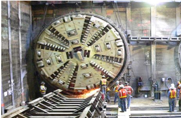
Tunnel Boring Machine
