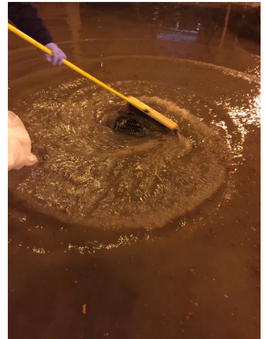
Mariachi Plaza Station Entrance by Bailey St.
