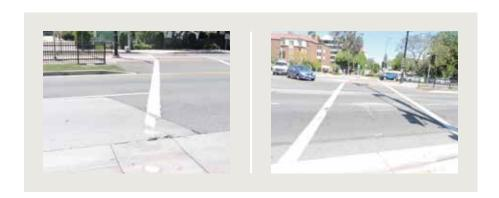
There are only fading white lines to mark the pedestrian crossing. There is no channelization to guide pedestrians through the crossing.
