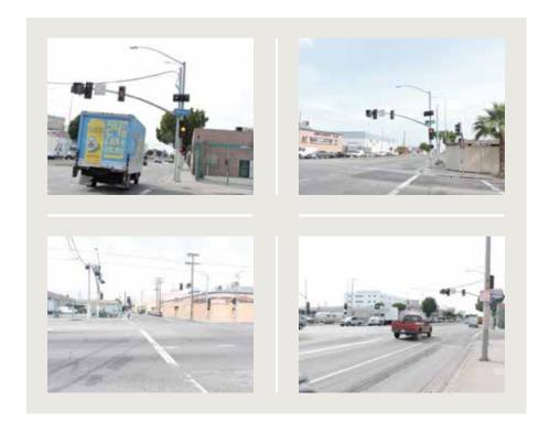
Traffic signals are provided at the intersection to control the movements of vehicles, trains and pedestrians. A multi-phased traffic controller controls traffic signal aspects as well as the bar signals for trains. Pedestrian signals are activated manually via push buttons.
