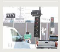
Traffic signals are provided at the intersection to control the movements of vehicles, trains and pedestrians. A multi-phased traffic controller controls traffic signal aspects as well as the bar signals for trains. Pedestrian signals are activated manually via push buttons.
