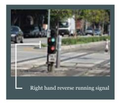
There is a lack of standards regarding the placement of wayside signals versus the Rail Operator's direct line of sight. Signal height, for example, varies from location to location and in some cases a signal is raised in an attempt to differentiate it from an adjacent signal. This condition was also observed by the APTA Peer Panel.
