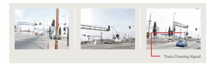
This intersection is equipped with basic crossing gates, flashing lights and bells for vehicles. There are no pedestrian flashing lights, gates or bells at this intersection. The only pedestrian crossing lights at this intersection are countdown lights that are manually activated by pedestrians.
