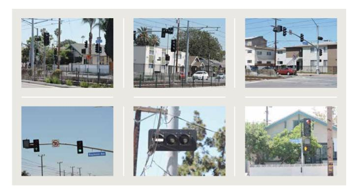
Traffic signals are provided at the intersection to control the movements of vehicles, trains and pedestrians. A multi-phased traffic controller controls traffic signal aspects as well as the bar signals for trains. Pedestrian signals are activated manually via push buttons.
